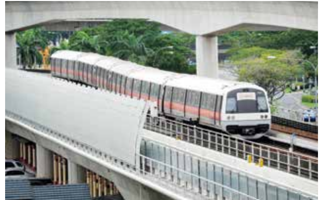
Noise barriers near Jurong East MRT Station
